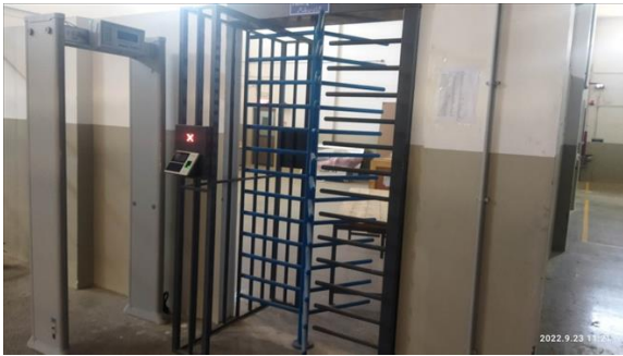
Packing Area (under constructoin)
